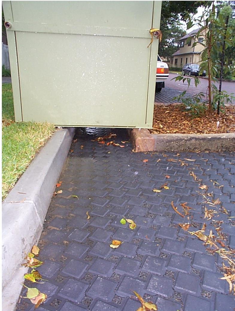
**Figure 4. The stormwater monitoring station at the gutter.**
