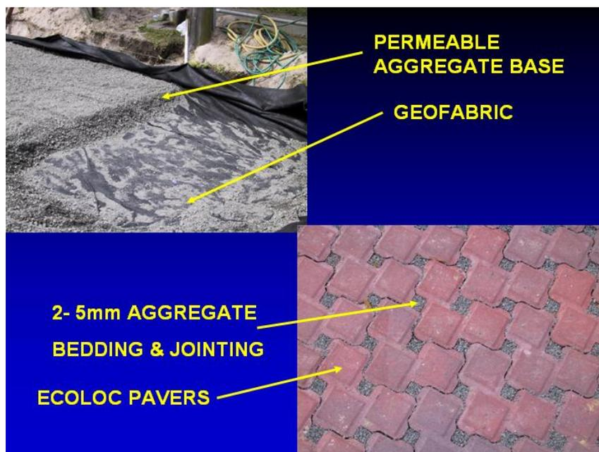
**Figure 1. Details of basecourse and surface construction.**
