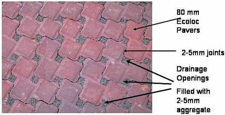
Figure 1. Typical Surface of a Permeable Eco-pavement (Smith Street, Manly)
