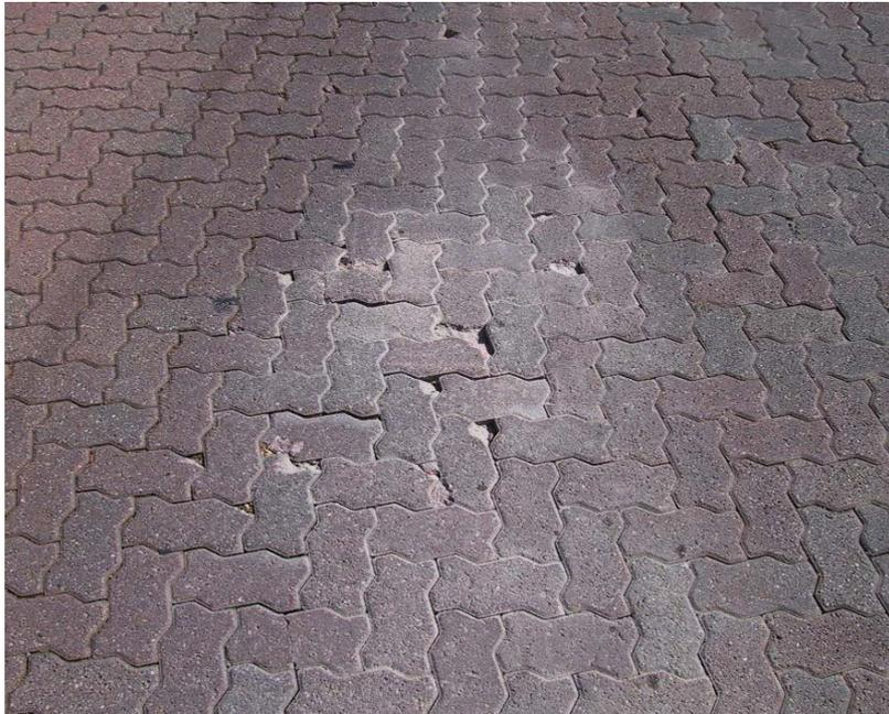
**Figure 3. Localised pavement damage showing loss of sand and chipping adjacent to Location 4**
