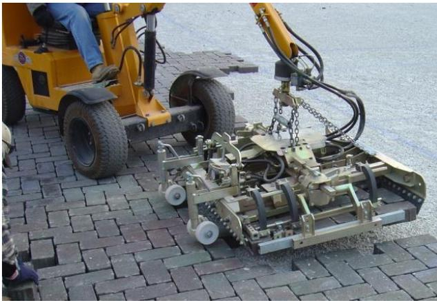
**Figure 9. Paver installation.**
