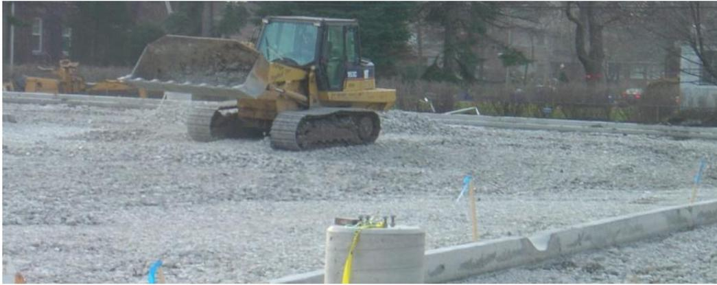
**Figure 8. Sub-base placement.**
