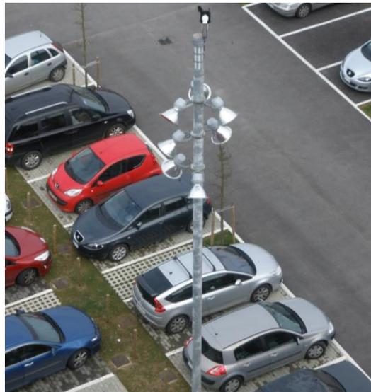
**Figure 4. Meteorological station placed on a stoplight of the experimental parking area.**
