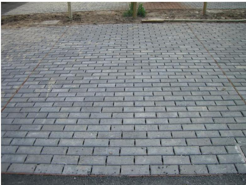
Figure 1. Pervious pavement surface of Aquaflow blocks.
