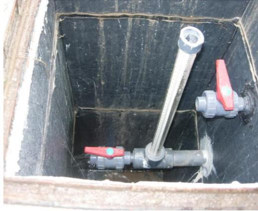
**Figure 3: Control manhole with the pipe connexions and the water level tube.**
