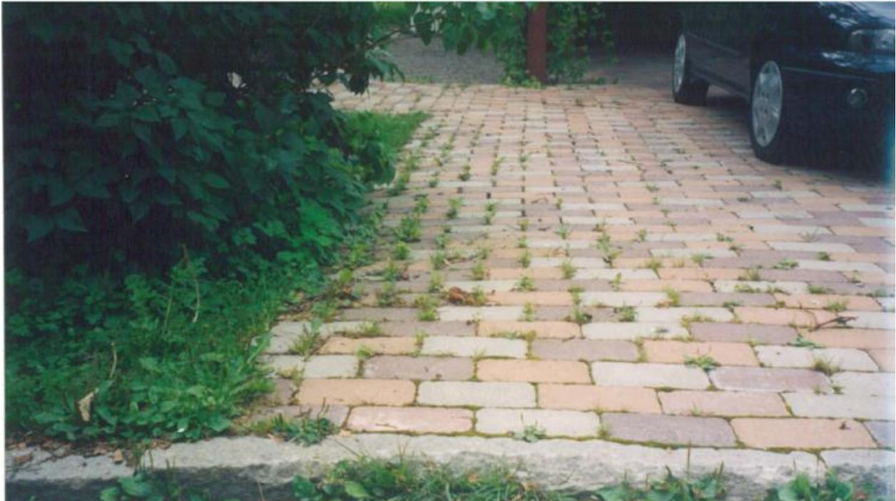
Figure 5. If edge restraints are missing, the lateral support will be poor. Photographer: 1<sup>st</sup> author.
