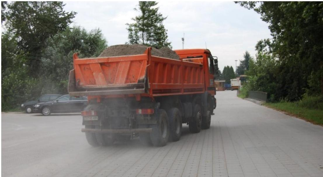
Figure 3. High axle load traffic on PICP.
