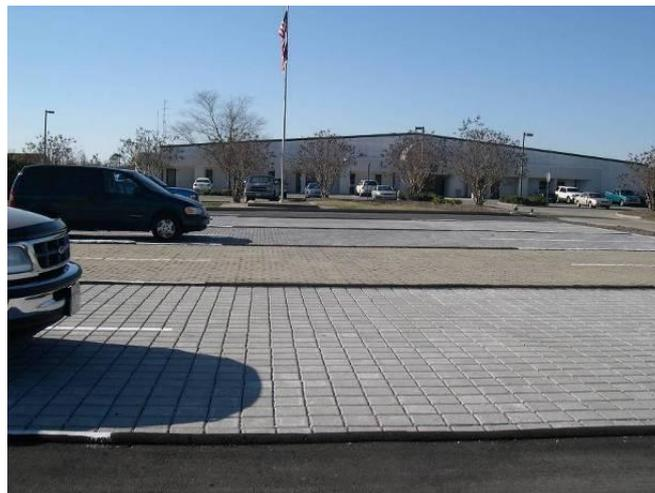
**Figure 1. Permeable pavement parking lot at the City of Kinston, NC.**
