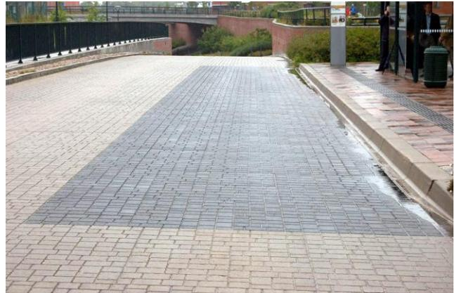
**Figure 2. Block pavement on a impermeable base layer (CTB) with bus traffic, three (3) years old (60 busses per day + public traffic).**
