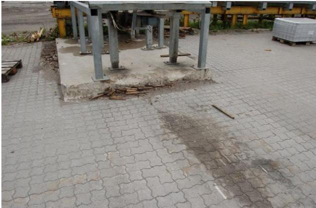
**Figure 1. Section of the first test site with the highest load concentration by forklifts with solid tires, (eight (8) years old, average 100 forklifts per day).**
