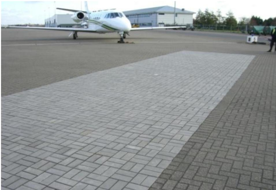
**Figure 6. Trial area of T & G units at RAF Northolt.**
