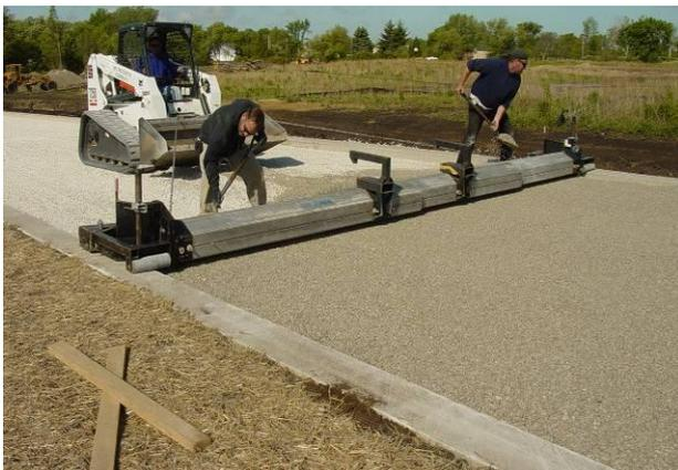
**Figure 11.** A mechanical screed relies on curbs or metal guide bars for creating a consistently thick PICP bedding layer.
