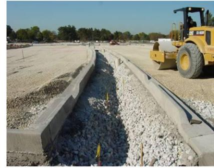
**Figures 8 and 9.** The depth of the concrete curb separating PICP from conventional pavement should extend the depth of the conventional pavement. Note the PICP in travel lanes in Figure 6 and PICP in parking spaces in Figure 7.
