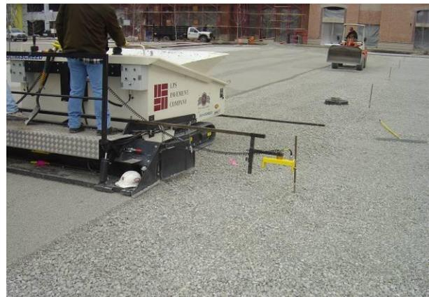
**Figure 12.** Laser guided screeding equipment adapted from the asphalt pavement industry can accelerate screeding of large PICP areas.
